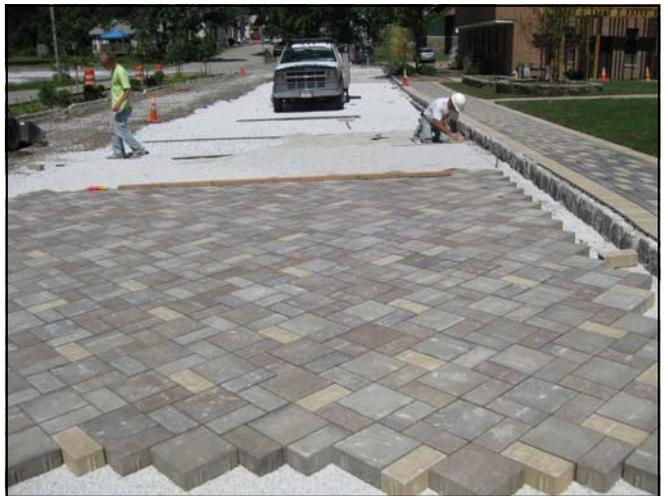
*At work on installing the pervious pavers.*
